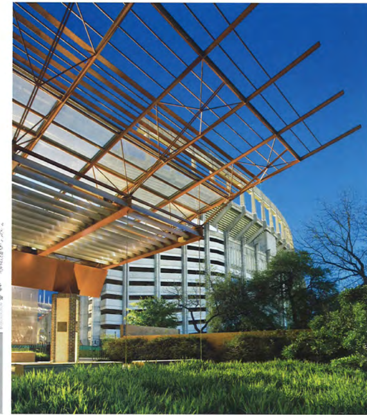
↑ | Close up view of the steel structure
