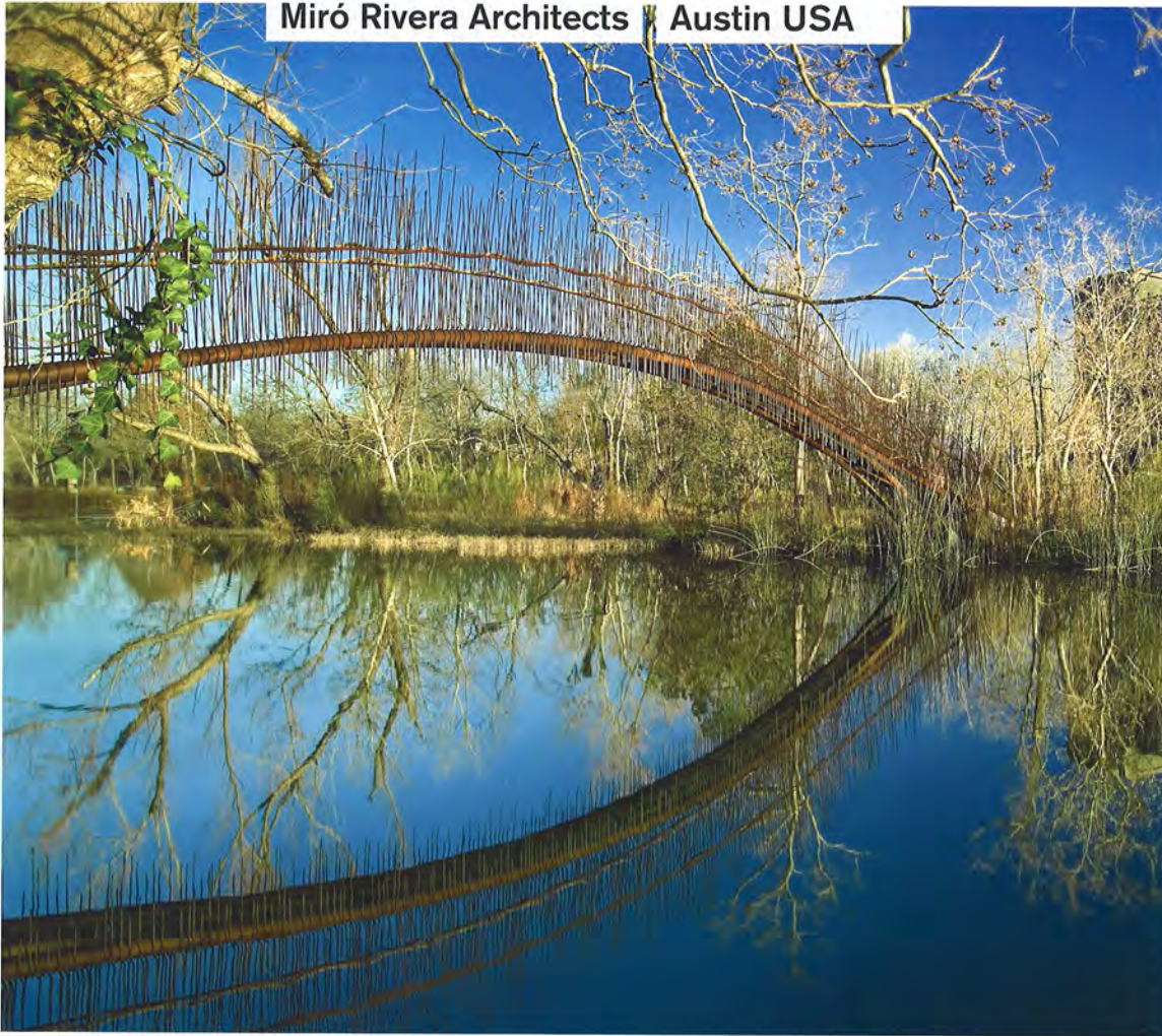
Pedestrian Bridge, Austin, Texas, USA, 2002–5. With a design inspired by the reeds that cover the lake, this pedestrian bridge is a light structure integrated in its setting. The bars/reeds intertwine at the abutments and “grow” over the bridge, camouflaging and turning it into a symbiotic, almost invisible link. To further integrate the bridge into its setting the steel is left unfinished, as are the rope handrail and the stone ramps.
